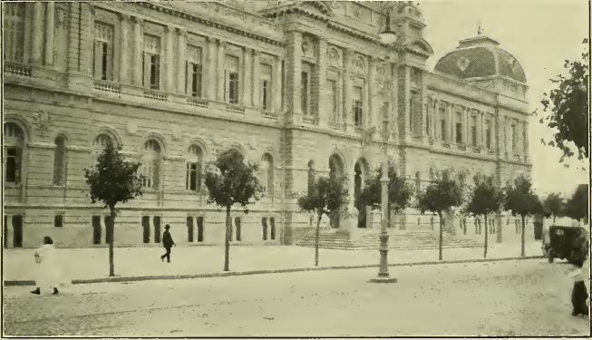
A. PRINCIPAL FAÇADE OF THE NEW UNIVERSITY BUILDING AT MONTEVIDEO.
